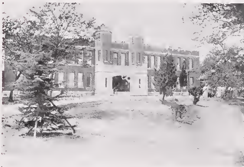
Main Building, Built 1931.
